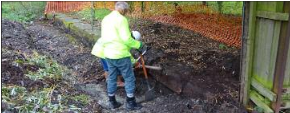
Exposing the wharf wall at Wappenshall
