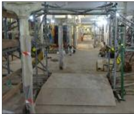
View along the ground floor of the Flaxmill
