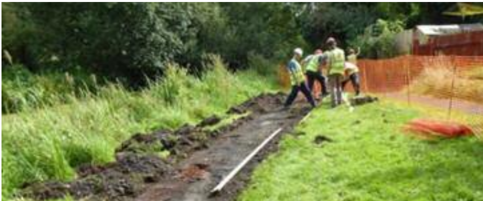
Work begins on restoring the Newport towpath
