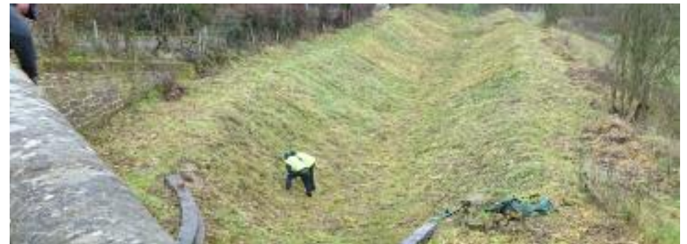
Forton with the undergrowth removed
