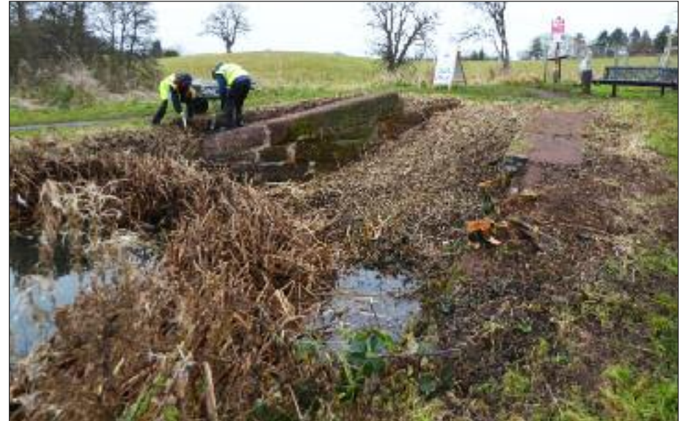
Clearing the stonework at the entrance to Meretown Lock
