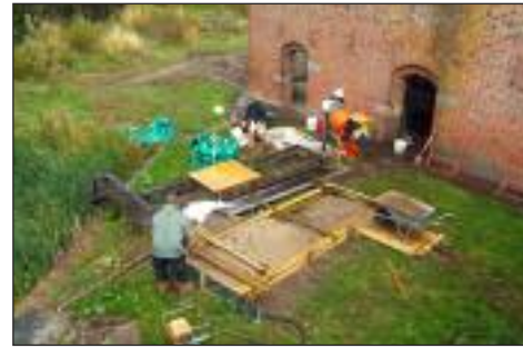
Laying the base
