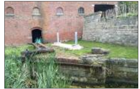
The gate waiting to be installed
