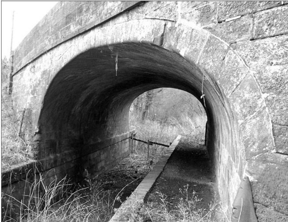
The Skew Bridge at Forton
