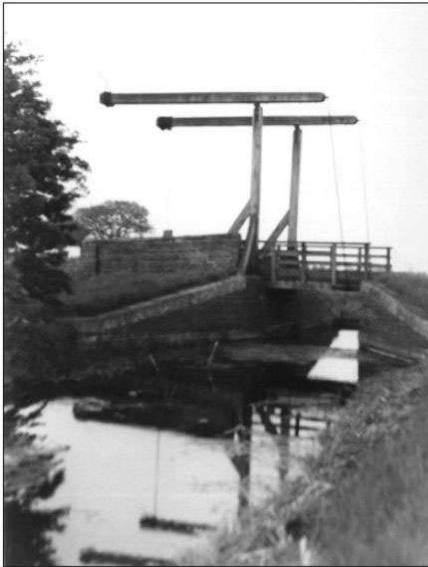
A Shrewsbury Canal lift bridge at Rodington
