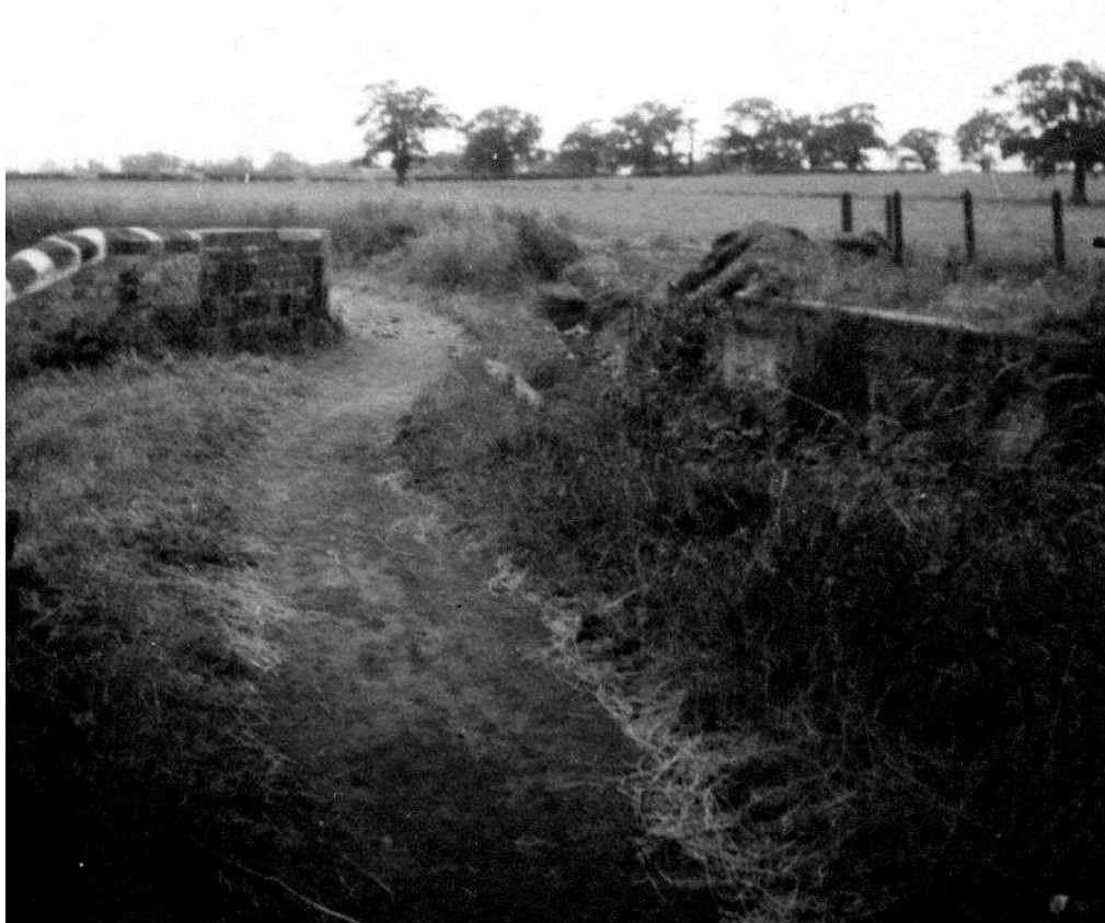
The path over Sundorne Aqueduct
