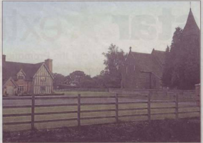
Church Farm and Withington Church are no longer connected by a lift bridge
