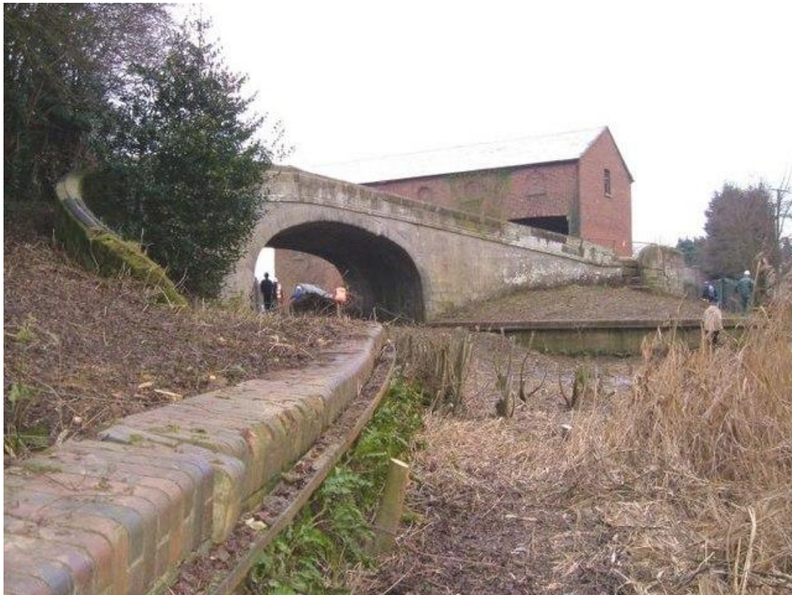
Unrestored West Basin, skew bridge and main warehouse (Photo by Roger Dean geograph.org.uk )
